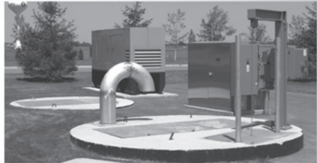
Lift Stations-New and Retro-fit Upgrades
